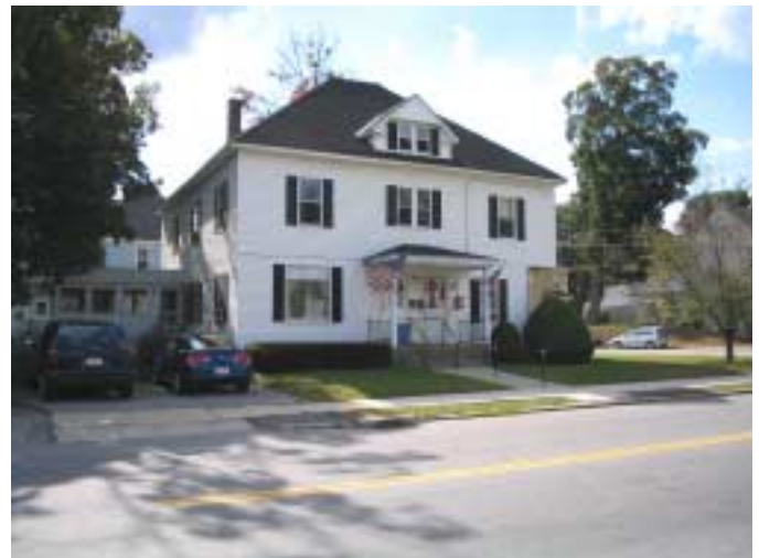
SCRRRI residence in Leominster where Paul Frain suffered neglect.
